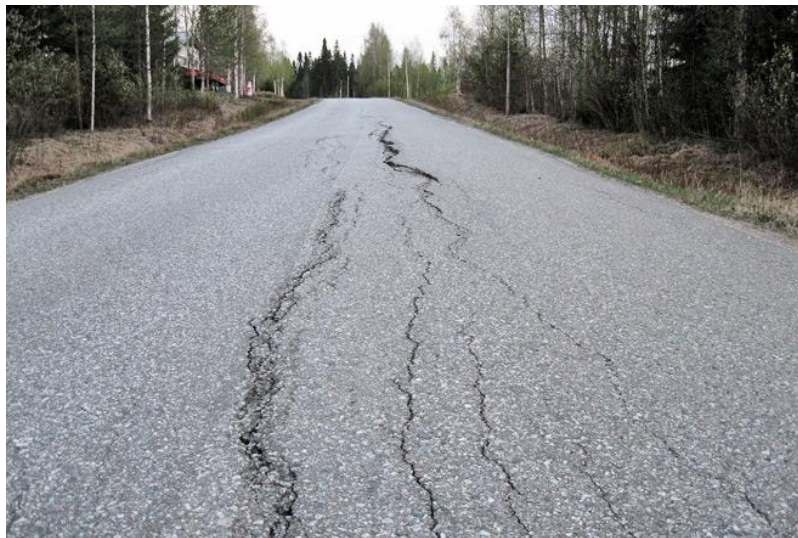
Fig.1. Shear cracks.
